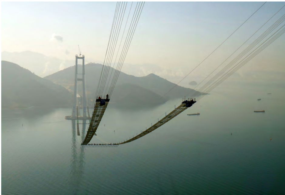
Yi Sun Sin Suspension Bridge, Catwalk Work, Gwangyang (photo: Si-Chul Kim)
