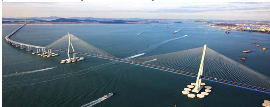
Incheon Bridge, Incheon
