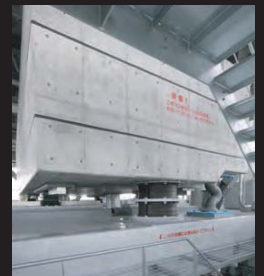
Roof Vibration Control
