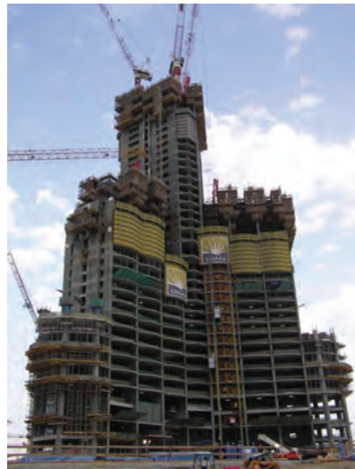
The Tower under Construction
