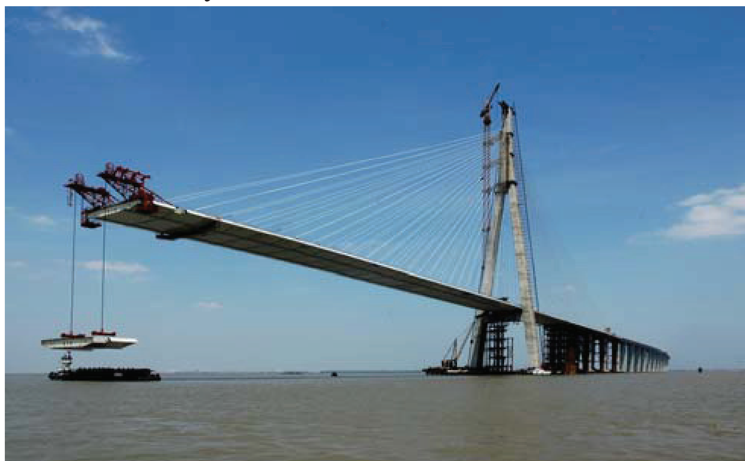
Fig.3: Erection of Box Girder
